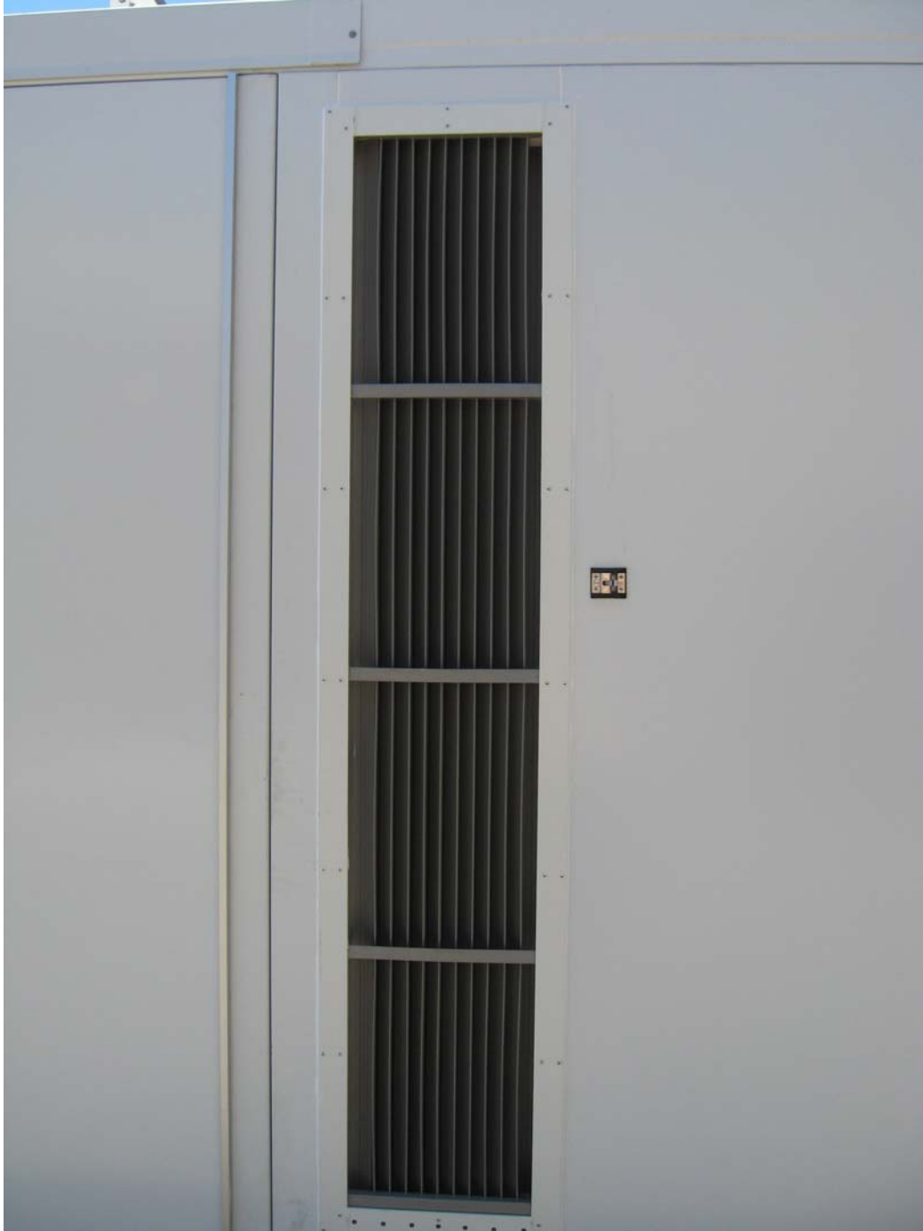
Moisture Eliminator Which has been installed on an Acoustic Enclosure
