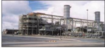
120MW gas turbine acoustic enclosures
